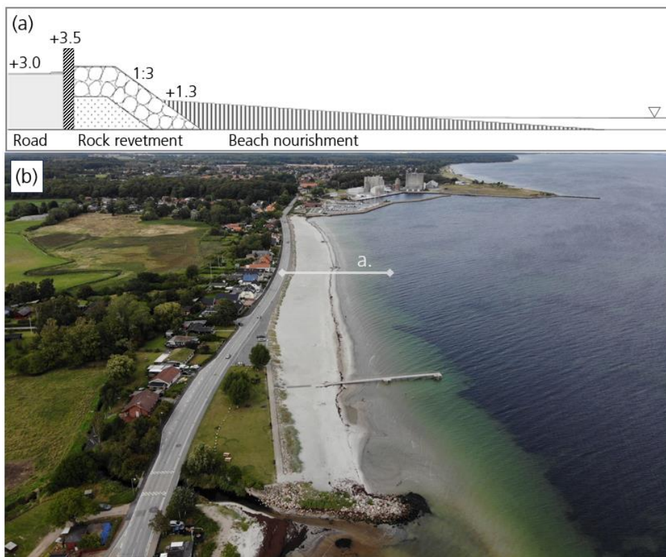
Figure 3.3: (a) Cross-shore schematic illustration of the combined coastal protection solution. (b) Overview of the coastal protection solution at Faxø Ladeplads, Denmark. The nourishment is placed between the harbour mole and the groin with the objective to reduce wave impact on the coastal road Strandvejen. Photo: Danish Coastal Authority, July 2021.
