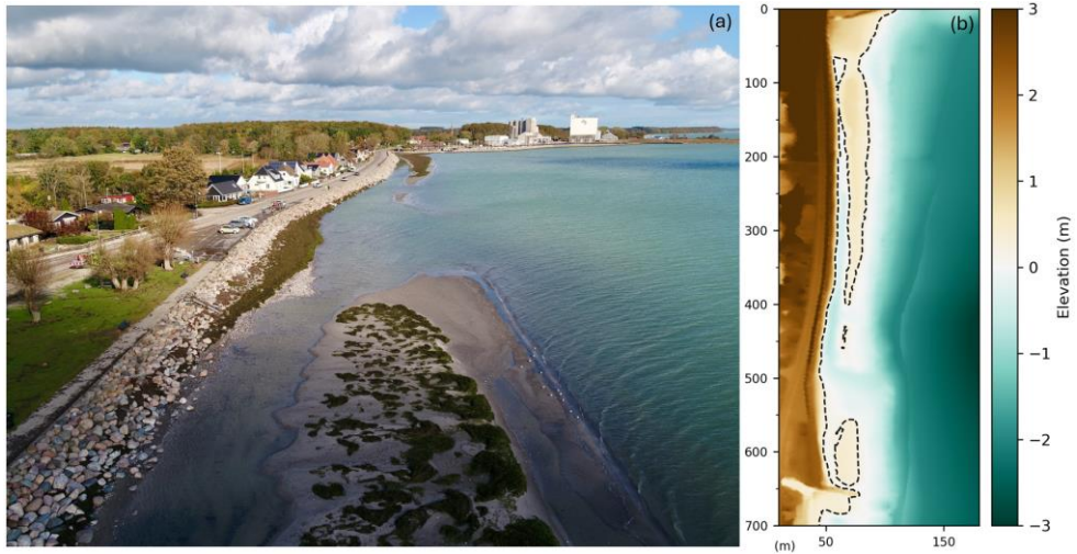
Figure 5.3: (a) Drone image to show an overview of the protection at the site after impacted by storm Babet (Photo: Gregor Luetzenburg, 23 October 2023), water level was +30 cm MSL. (b) Post-storm DEM, black dashed line corresponds to +30 cm MSL and thereby highlight the emerged areas shown in (a).
