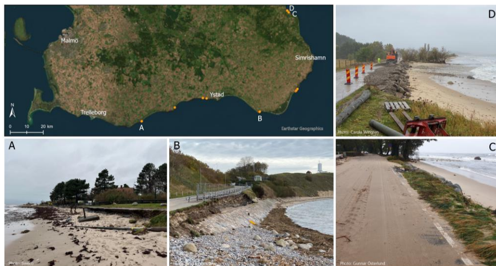
Figure 5.5: Documented damages to roads caused by storm Babet in October 2023. (A) Beddingestrand - Private owned road damaged by storm erosion, photo: Sweco. (B) Kåseberga - State owned road undermined due to storm erosion following wave runup on the structure, photo: Bradley Goodfellow. (C) Kivik – road impacted by flooding and overwash, photo: Gunnar Österlund. (D) State owned road between Kivik and Vitmölla damaged through storm erosion, photo: Carola Wingren.
