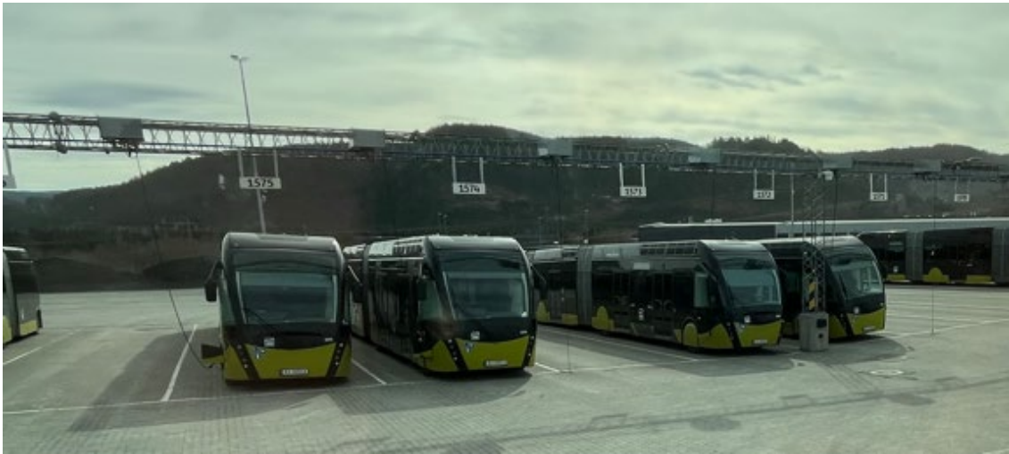
Figure 3. Buses charging at the depot in Trondheim
