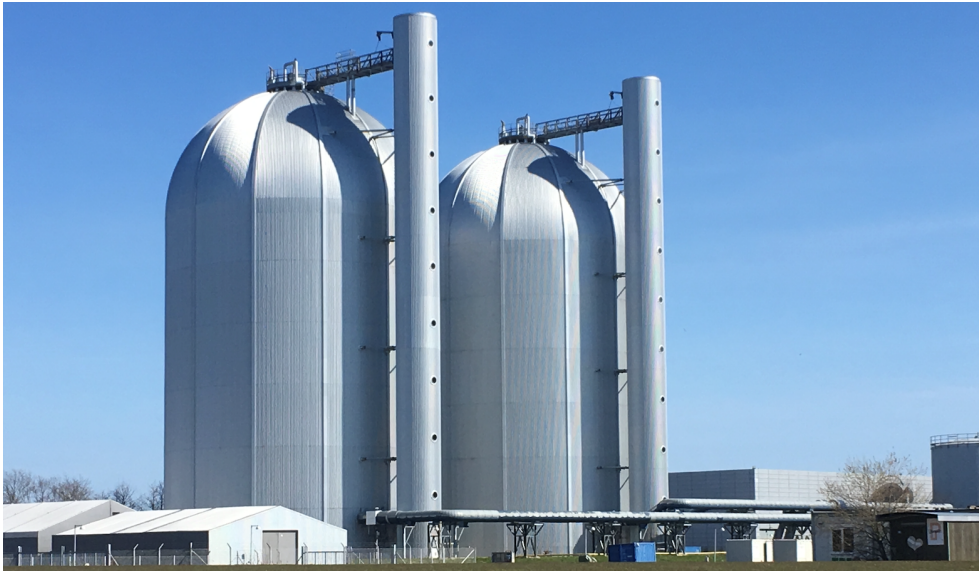
Figure 3.9: Water tanks in Avedørværket, Denmark, each holding a volume of 24 000 m 3 (Andrews et al., 2012, page 71). Source: The author.
