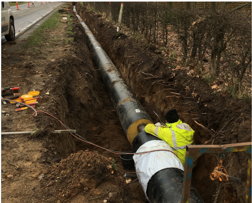
Figure 3.1: Welding of a twin pipe in Gelsted, Denmark. Source: the author.
