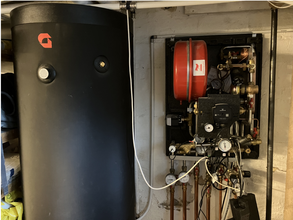
Figure 3.3: Substation with indirect connection for space heating and preparation of domestic hot water with accumulation in Copenhagen, Denmark. Source: the author.
