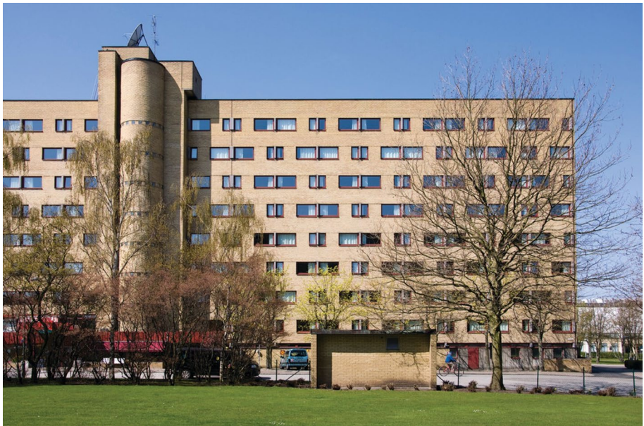
Fig. 9 Piræus, Malmö, designed by Bengt Edman. The single stairwell serving the entire building is clearly demarcated in the façade (Unknown photographer, by courtesy of Malmö City Archive)
