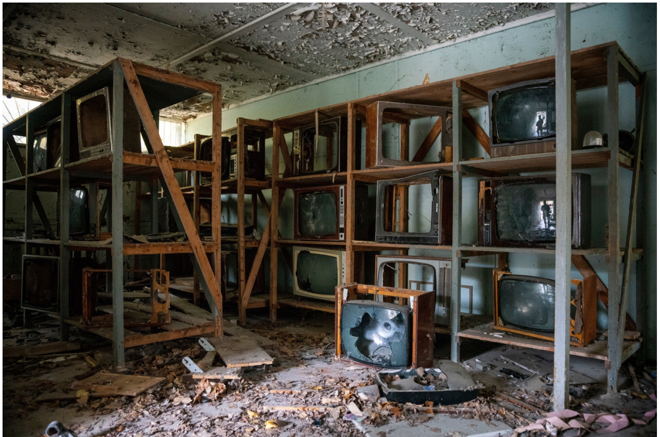
FIGURE 37 In an abandoned shop in Prypiat. Scavengers have broken the televisions for the scrap metal to sell on the black market. Photo by Carsten Olsen, 2021.
