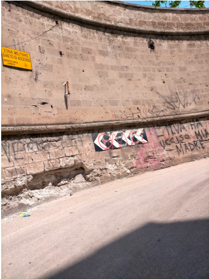
Figure 3 The Arsenal wall. Photo by the author.
