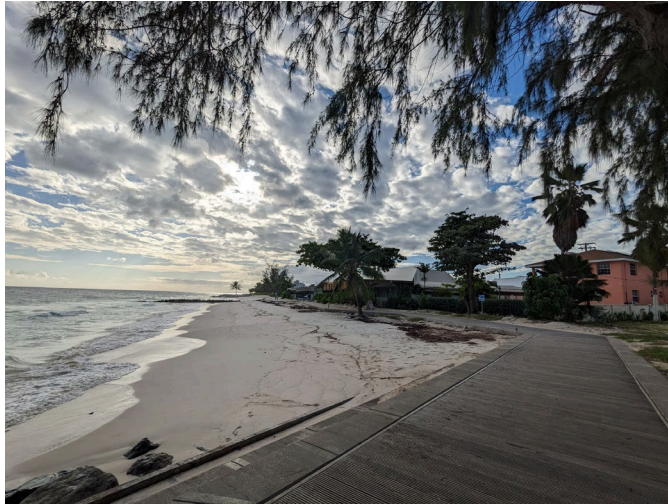
Picture 05. Rock armour revetment and boardwalk along the southern coastline of Barbados, the adaptation project referred to by the interviewee.
