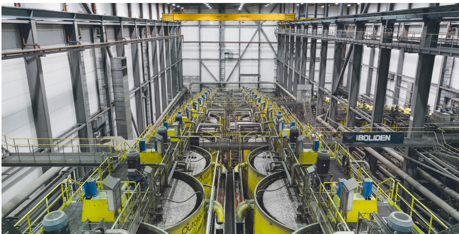
Photo of the flotation series in the Aitik concentrator, located near Gällivare, Sweden. Photo credit: Jonas Westling.
