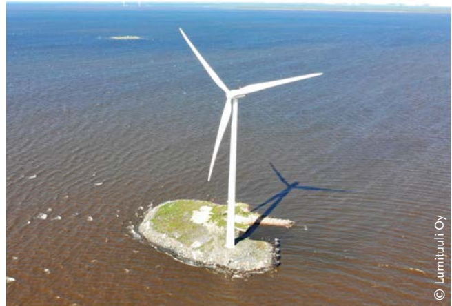
FIGURE 3: 2 MW wind turbine in Lumijoki, Finland, owned by Lumituuli Oy, Finland's first and largest consumer-owned wind power company.
