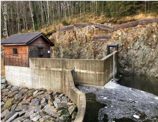
FIGURE 2: Inlet to the small hydro power plant Åkra in Kvinnherad, Norway. Owner Vika AS. Effect: 4.1 MW. Fall height: 401 meters.
