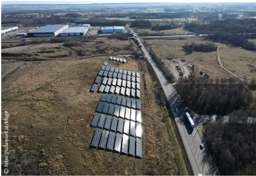
FIGURE 4: PV park Solar Park in Helsingborg, Sweden.
