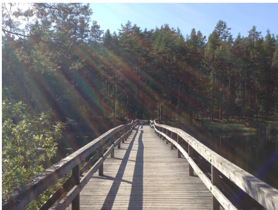
Figure 1: View of the bridge where I met Matti, with bench alcove further along and to the left (August 2023)
