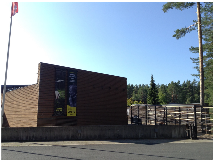
Figure 5: View of the museum building from the road (August 2024)
