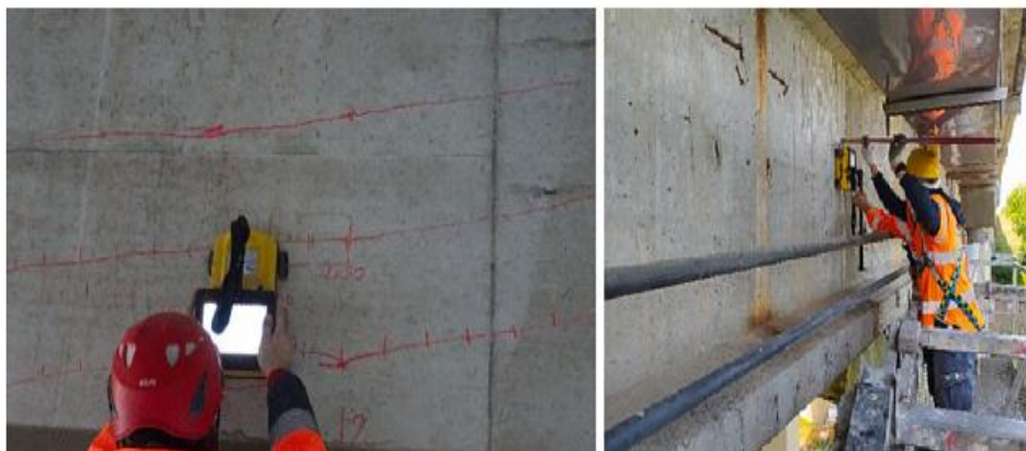
Figure 5-2: In situ execution of GPR tests.
