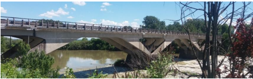
Figure 8-22: Picture of the studied bridge
