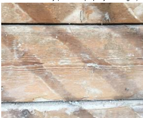
Figure 4. Exposed timber of an historical bole house in Visby (the same property as in Fig. 2 and 3) after the wooden slats and lime plaster had been removed.
