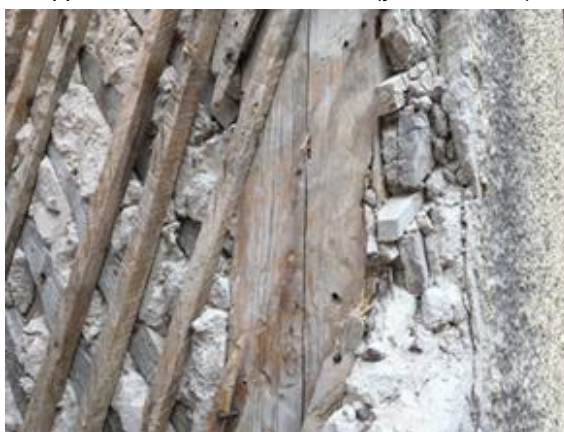
Figure 2. Exposed lime plaster embedded in diagonal wooden slats on another property in Visby. Here the lime and wooden slats were removed in order to apply mineral wool insulation with the goal to improve energy efficiency.
