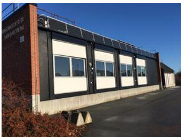
Figure 7. Two façade sections will be replaced with "historical" timber façades.
