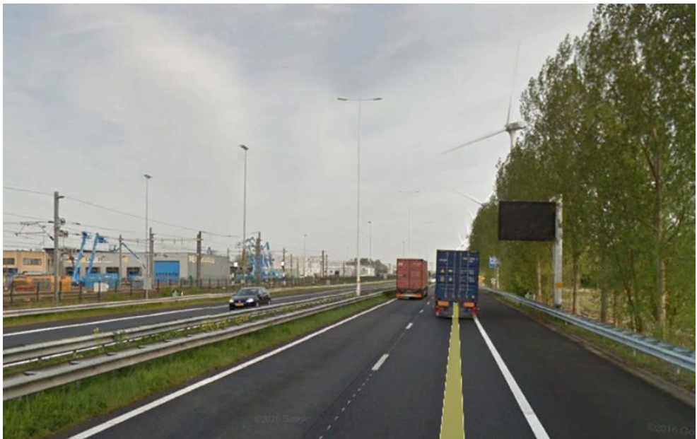
Figure 36 – Research location. Street view near camera 1 after construction of wind turbines (image adopted from Google Street View).
