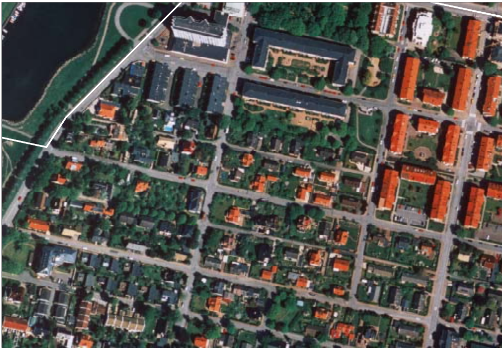
Figure i:36 In Sibbarp there are several morphs, such as lamellar yard shapes in the northeast and row house blocks in the northwest.
