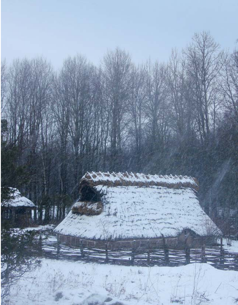
Figure 37. The longhouse from the Bronze Age. Sten Tesch's reconstruction of house B14:VIII from Köpingbo, southern Sweden, built on The Ekehagen Ancient Village site. Today, 20 years after it was built, the house is still standing and works well (2015). The room division is similar to that at Pryssgården house 172. The house had a package of clay wrapped in a textile (which left imprints in the clay) and was kept in a so-called storage pit well protected from frost. Already in 1984 Tesch reported it as a prepared clay package that was being stored for use in the farm's pottery production (Tesch 1993:165), an early artisanal-perspective interpretation. Photo Henning Cedmar Brandstedt.
