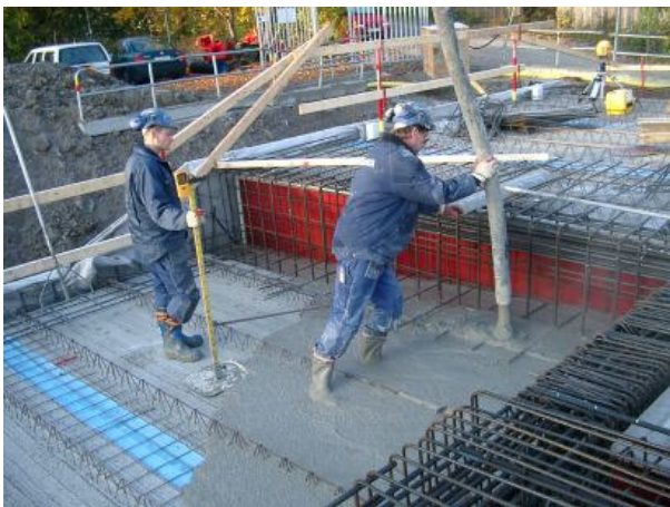
Figure 4.4 Casting of slab using SCC.
