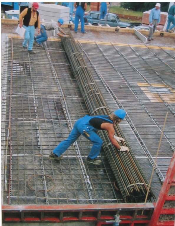
Figure A.19 The BAMTEC-system is an example of competitive reinforcement solution (Fundia, 2002).
