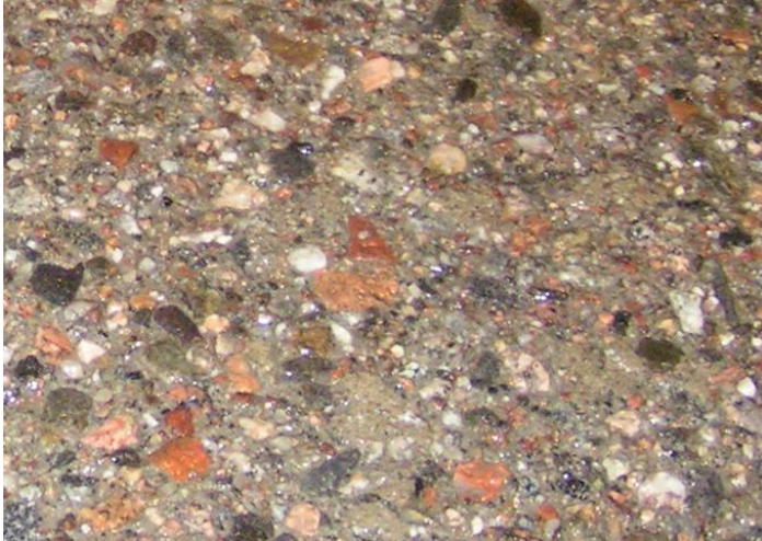
Figure 5.12 Increased roughness and presumptively increased strength as well of the concrete surface of the first specimen through utilisation of exposed aggregates.
