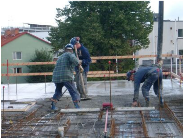
Figure 4.3 Casting of slab using traditional concrete.
