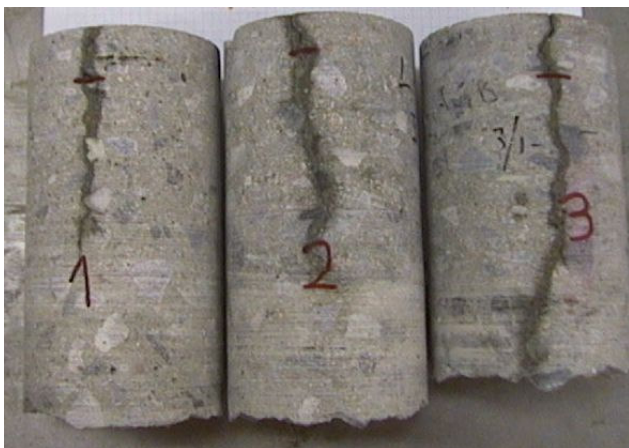
Figure 4.17 Drilled cylinders taken out from slabs cast with SCC showed the depth of cracks due to plastic shrinkage.
