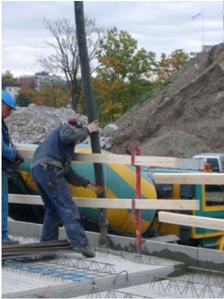
Figure 4.10 Placing of SCC in walls.
