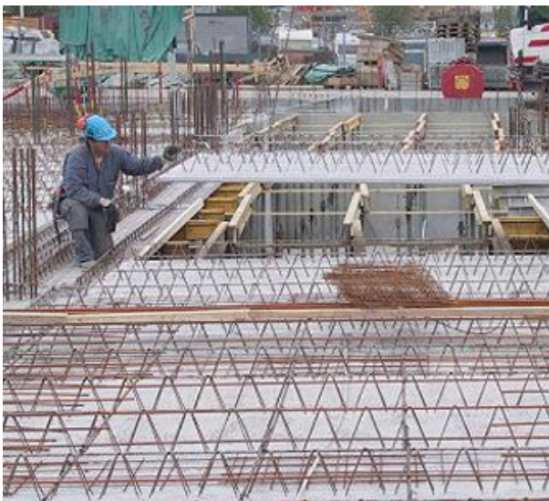
Figure 2.2 Precast formwork system for permanent use, i.e. Filigran type of formwork, is a common method in combination with ready-mix concrete cast in-situ. Photo taken from ‘Betongbanken’, ( see SFF, 2007), a planning tool including experience from use of ready-mix concrete.
