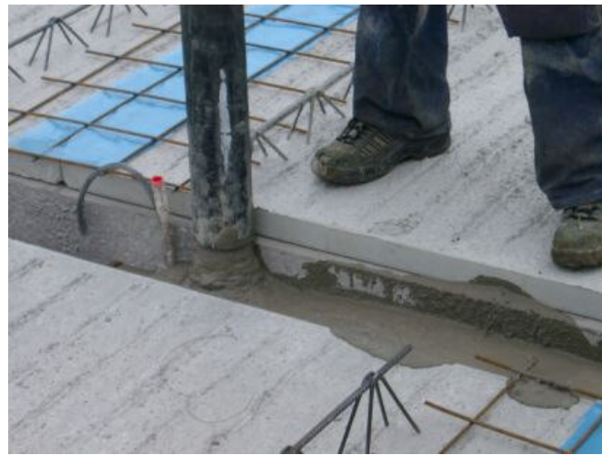
Figure 4.11 Placing of SCC in walls by using pump (close-up).
