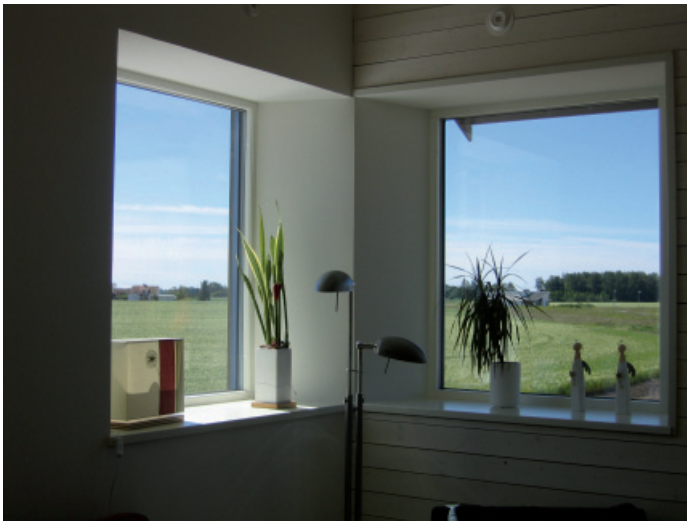
Figure 5.26 Non operable windows on second storey, left window facing east.
