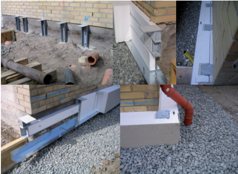
Figure 6.14 Thermal bridge insulation around foundation slab construction.
