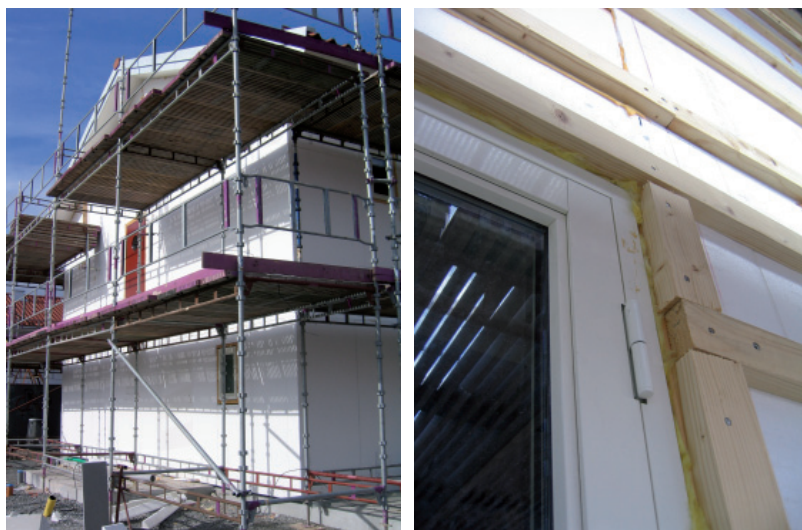
Figure 4.8 Outer walls covered by expanded polystyrene insulation (EPS).
