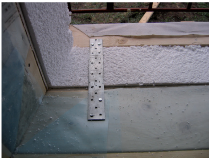
Figure 5.15 Nail plates in window openings.
