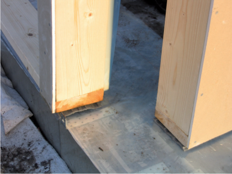
Figure 5.7 Moisture protection of wooden beam construction.
