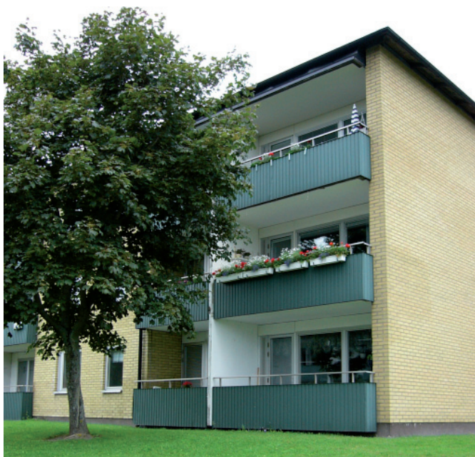
Figure 6.7 Original balcony construction inset into the apartments.
