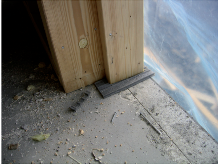
Figure 4.9 Moisture protection below the wooden sill construction.
