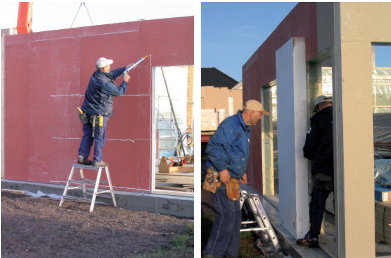
Figure 5.8 Polystyrene glued on the gypsum board.
