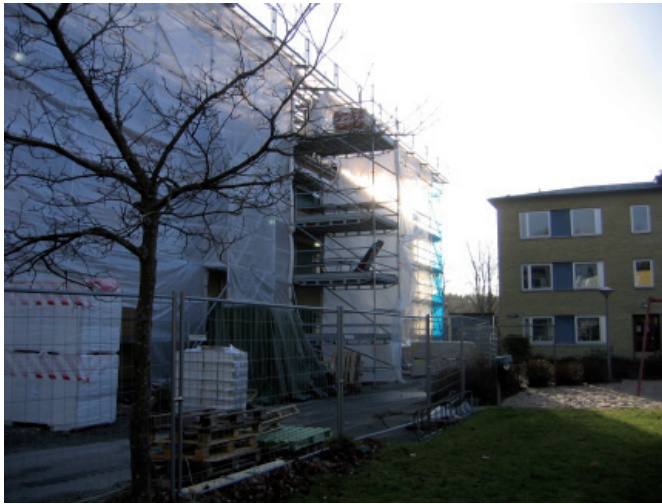
Figure 6.12 The demonstration building covered during renovation.
