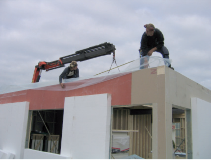
Figure 5.10 Floor mounted on top of the walls with careful folding of the plastic foil.
