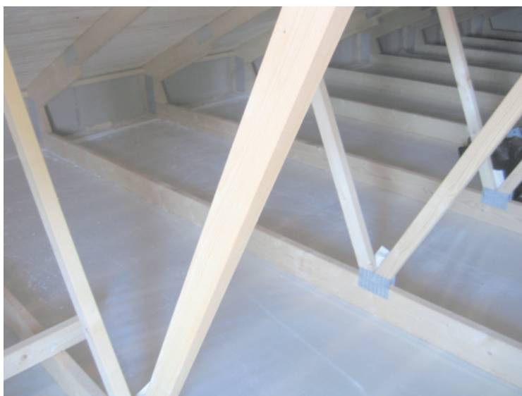
Figure 4.10 The attic, before the insulation was put in place.
