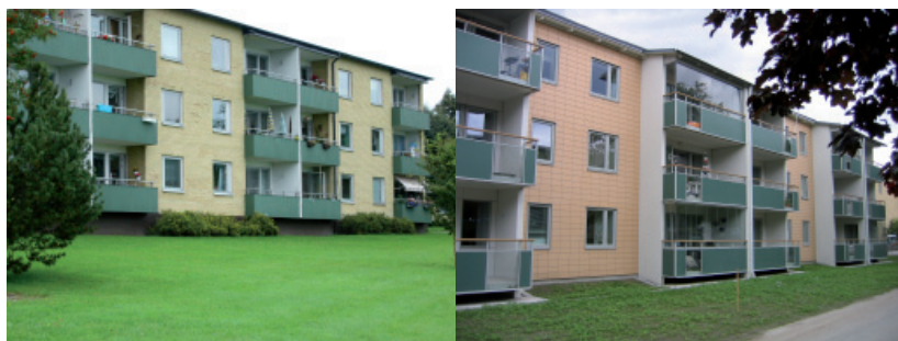
Figure 6.22 Long side façade with balconies before (left) and after (right) renovation.
