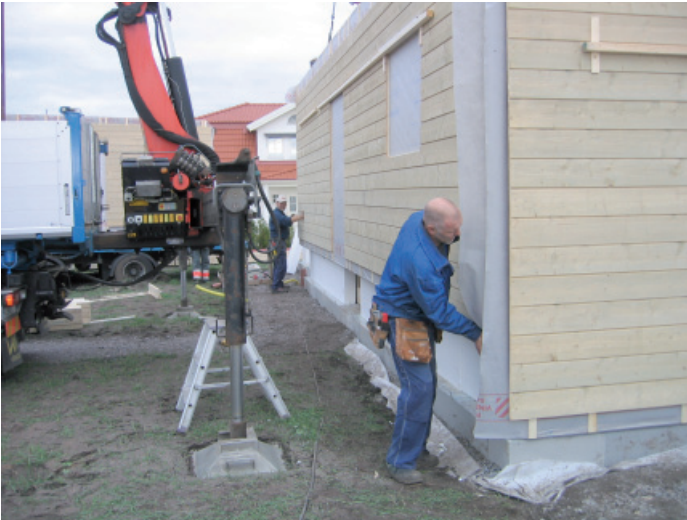
Figure 5.11 Outer wall slab mounted on the outside of the EPS insulation.
