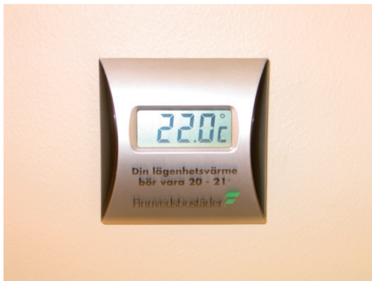
Figure 3.15 Display showing the temperature in each apartment.
