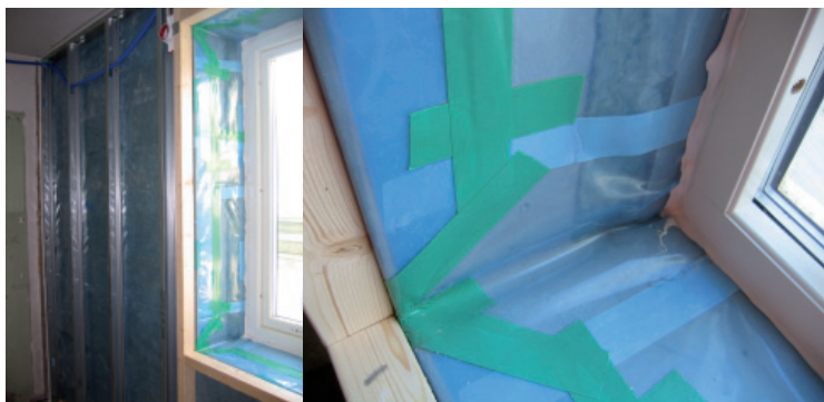
Figure 6.25 The sealing of the window sills.
