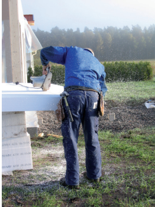
Figure 5.9 Polystyrene sawn up on site.
