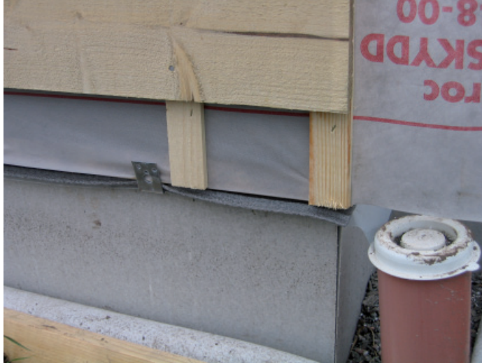
Figure 5.12 Lowest wooden panel detached to facilitate the mounting process.
