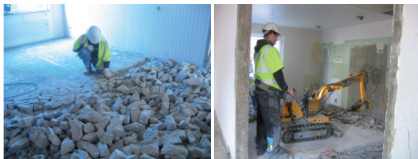
Figure 6.13 Removing the top layer concrete on the ground floor in Brogården.
