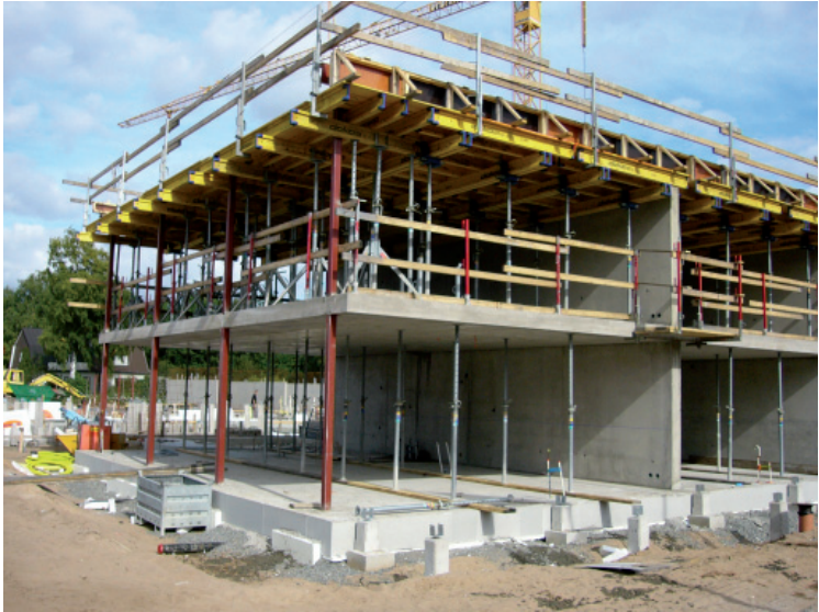
Figure 3.7 Concrete construction cast on site.
