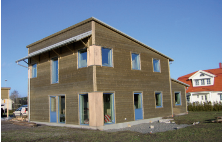
Figure 5.27 Lack of solar shadings on eastern façade.
