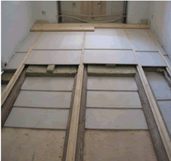
Figure 4 A Danish renovation project, before and after. Photo: Jens Holger Rindel.
