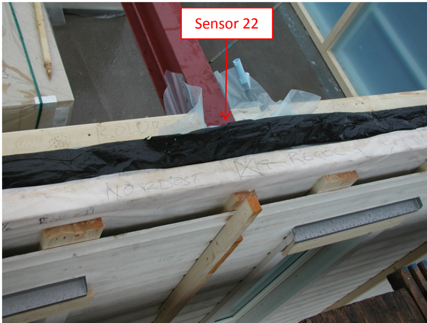
Figure 7.22.3. Location of the studied position before the sensor, the iron beam, the slab and the wall on the second floor was mounted.
