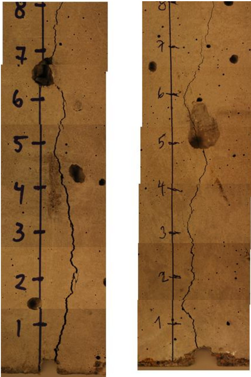
Figure 7.1: Photography of cracks before exposure. 75 mm cover. cm-scale indicated.
