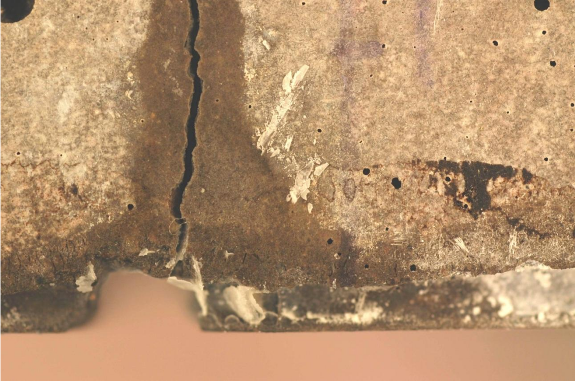
Figure 12.10: 0.4 mm sealed crack after 1 year permanent immersion in sea water. Test series 5, specimen S275-4-1-1.
