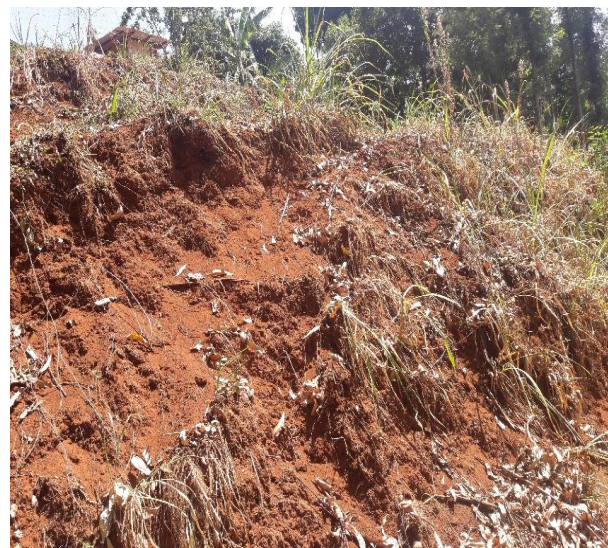
Figure 7. Degraded grass terrace in Gatura village.
