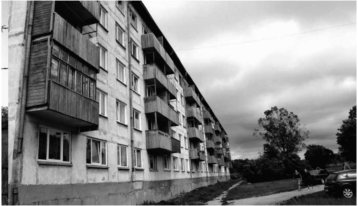
Paldiski – house with wooden balconies
