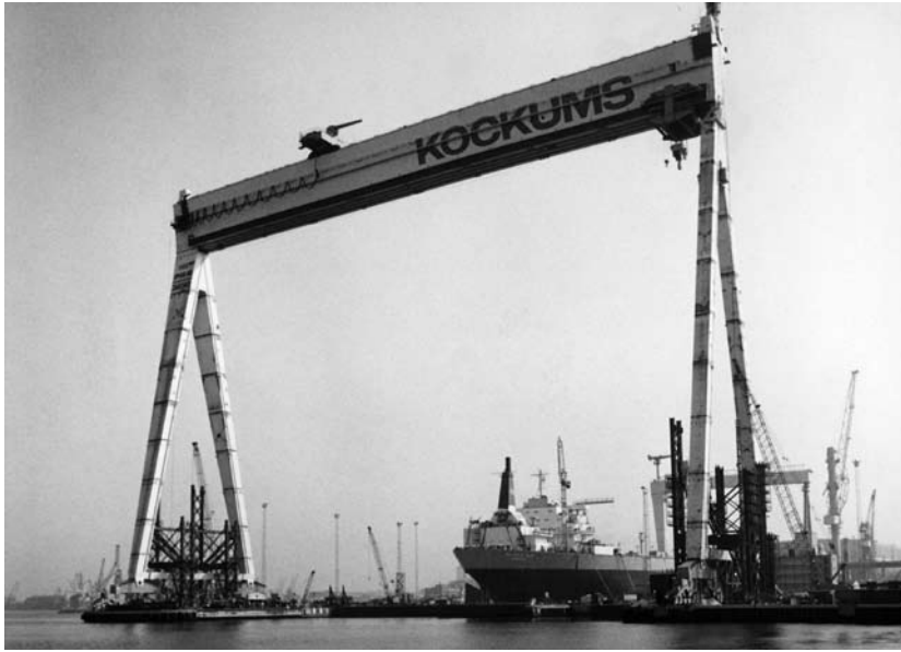
The great gantry crane at Kockums inaugurated in early 1974. ©Kockums mekaniska verkstad/Malmö Stadsarkiv.
