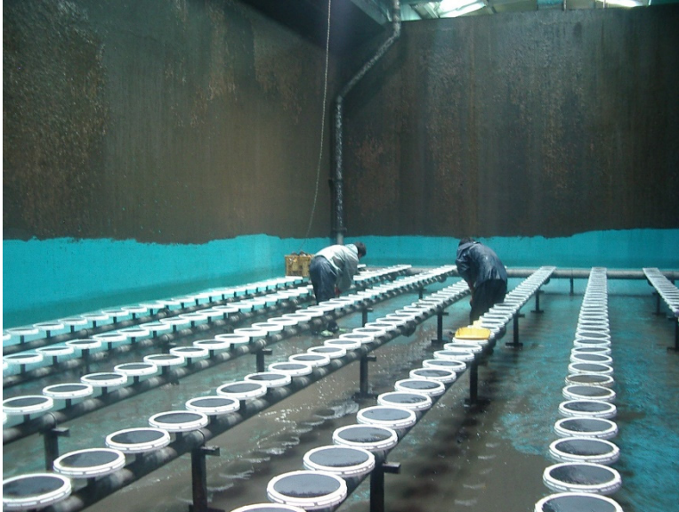
Figure 14 Picture of a bubble column installation in South Korea. Photo by PAOR CO., Ltd. (reproduced with permission).
