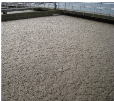
Figure 24 Aerated zone of untreated line at Öresundsverket WWTP
