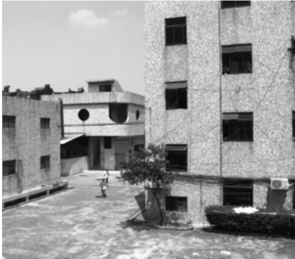
Dormitory buildings, Dongguan. Photo: Nlcnet.org
