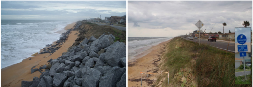
Figure 41: Left: Looking South along SR A1A in Flagler Beach showing actual conditions without USACE project in January, 2014. Right: Conceptual rendering of post-project conditions created by the USACE showing the proposed 10 foot dune extension. Sources: Left, Author's Photo, 2014; Right, image courtesy of Flagler County Engineering Department.
