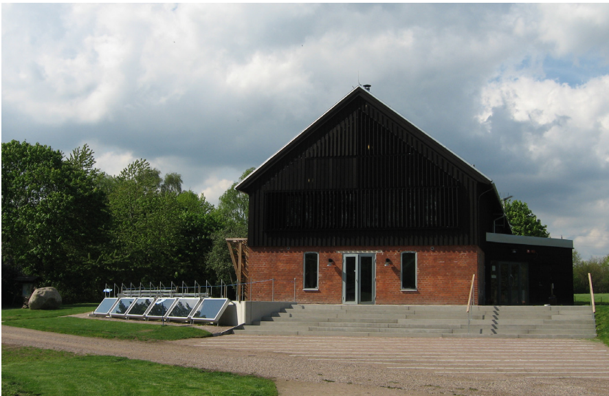
Figure 3.7 The solar collectors at the Fulltofta Nature Centre are mounted on the ground in order to give a signal to the visitors about the environmental concern of the building. This exhibition building is heated with solar collectors and ground-source heat pump. During winter time, wood is also used in a stove.
