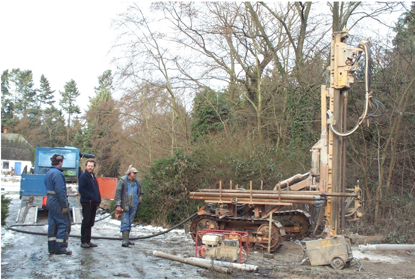
Figure 5.2 Drilling a borehole to a single family dwelling.
