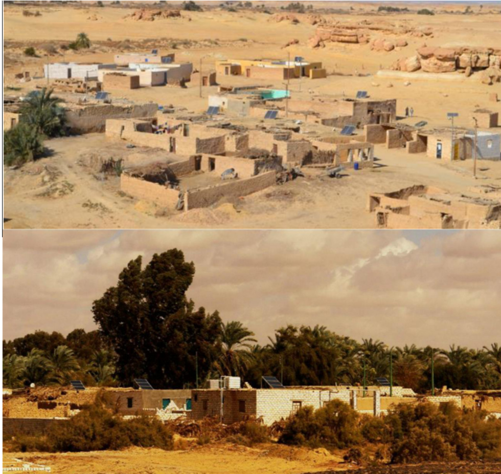
Fig. 1. A cluster of vernacular buildings in El-Gara, Siwa Oasis, Egypt (upper photo) and El-Heiz, Baharia Oasis, Egypt (lower photo) after the provision of the PV units.
