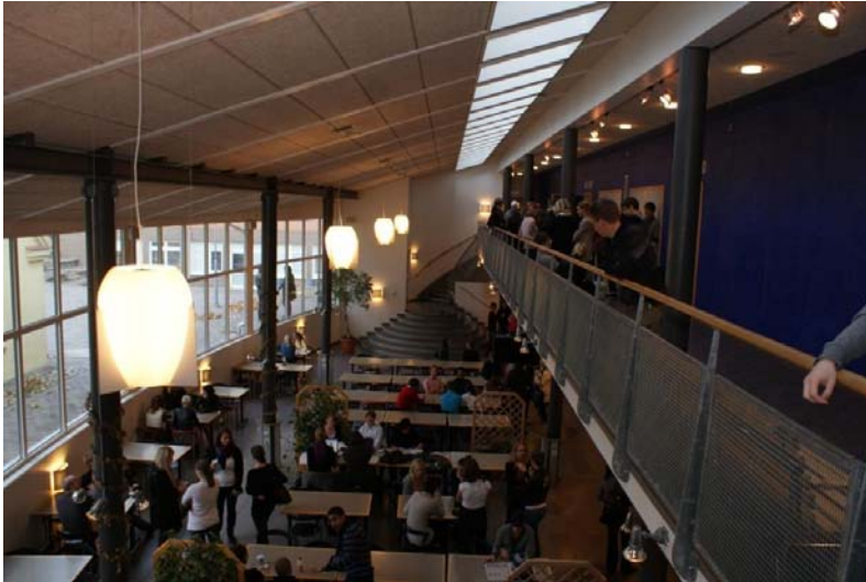
Figure 4. View from first floor, staircase 1. On the right you see the emergency exit of the first floor that is a part of the atrium and where occupants can be exposed to fire gases when a fire starts on the ground floor.
