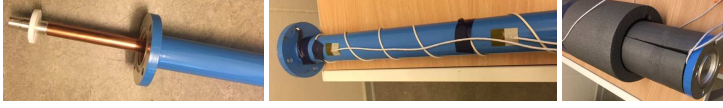
Fig. 1: Phase reference line of copper (left), heating cables and temperature sensors attached (middle), and insulation applied (right).
