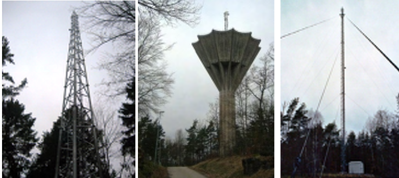
Pictures: To the left, a 3G tower in Gammalstorp, Blekinge. In the middle, a telecom mast on water tower in Bräkne-Hoby, Blekinge. To the right, a mast with tech shed in Äryd, Blekinge.
