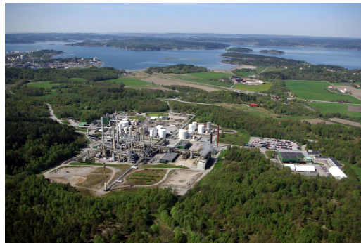
Figure 1.1 A process industrial site located in Stenungsund, Sweden.
