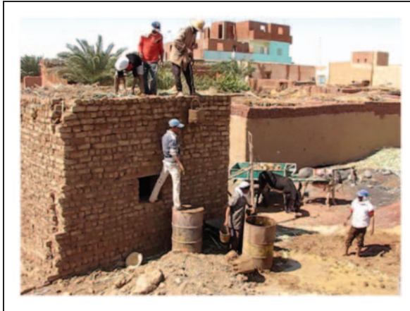
Figure 10. Applying the mud brick and the mortar layers.
