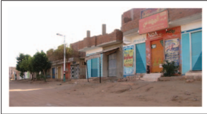
Figure 2. The new concrete urban pattern surrounding the periphery of Balat.
