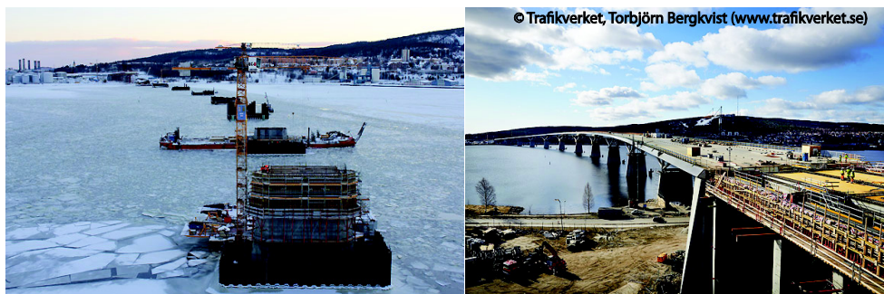
Figure 4.2 Bridge in central Sweden where sheet piles for drainage were also used as support piles
