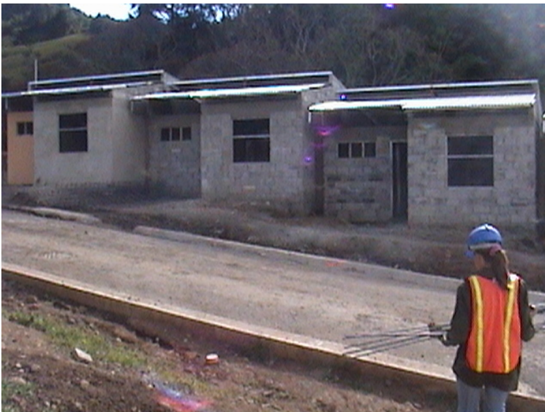
Figure 3: OSHH Project Nuestra Señora del Carmen, Costa Rica Source: Israel Figueroa, Civil Engineer, FUPROVI, 2006
