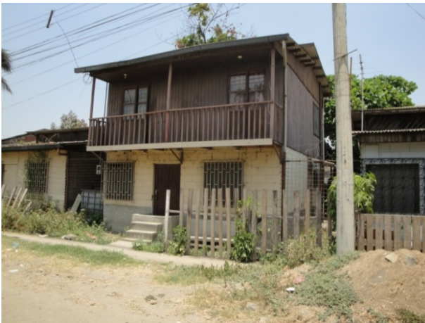
Figure 7. Prototype of the first housing typology showing that this typology could be extended vertically through self-construction of a second wooden floor. Photo: Ivette Arroyo, 2009
