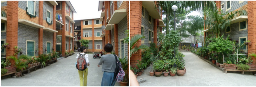
Figure 4.2 Taguig project is the first medium-rise building for OSHH implemented by Habitat for Humanity Philippines, households and volunteers. A three storey building in which each apartment units consists of two levels; the first level is for living and wet chores; the second level provides space for a loft for sleeping. Photos: Alvaro Vásquez-Esparza, Field trip to The Philippines 2011
