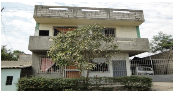
Figure 9. New housing replacing second housing typology in phase 7 with reinforced concrete structure and masonry block walls. Photo: Ivette Arroyo, 2009
