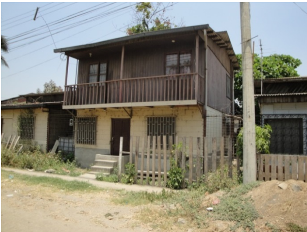
Figure 7. Prototype of the first housing typology showing that this typology could be extended vertically through self-construction of a second wooden floor. Photo: Ivette Arroyo, 2009
