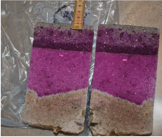
Figure 2.7. Core 5: Ground floor, painted surface.
