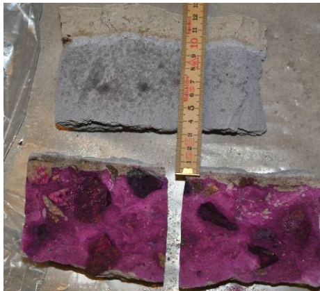
Figure 2.12. Core 8: Inside of external wall.
