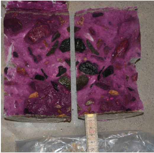
Figure 2.2. Core 2: Inner wall.
