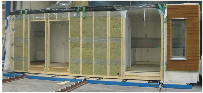
Figure 2.2: A TVE ready for transportation to the construction site.
