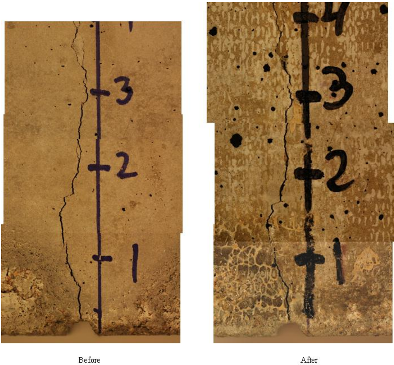
Figure A1.9: Water suction from the un-cracked side. Crack width 0.2 mm. Cover 75 mm. Specimen H75-2-3-2
