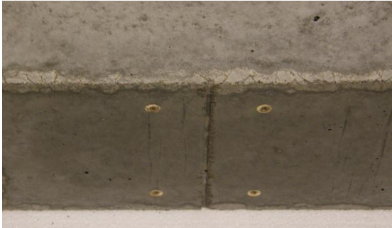
Figure 5.1: Cast-in nuts for mounting two extensometers across the notch.
