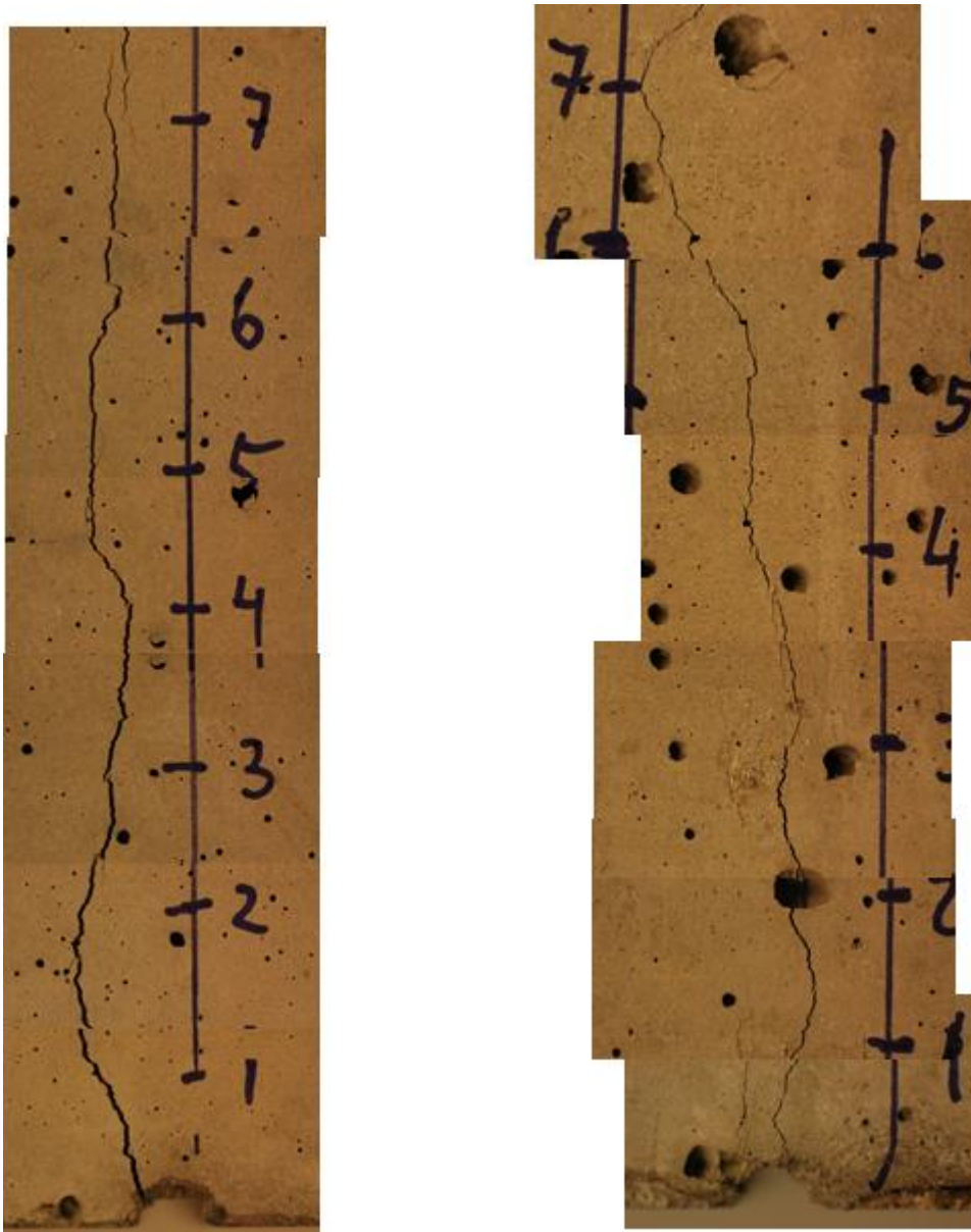
Figure 7.1: Photography of cracks before exposure. 75 mm cover. cm-scale indicated.
