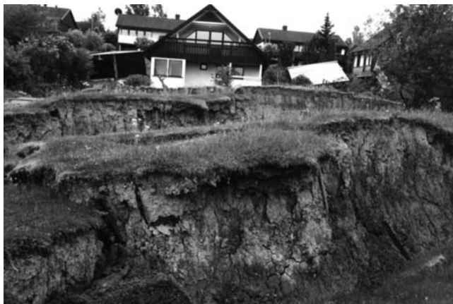
Fig. 7. Photograph of residential area in Vagnhärad after slope failure within Trosa River Valley in 1997 (photographer: Jan Lindgren, Swedish Geotechnical Institute)
