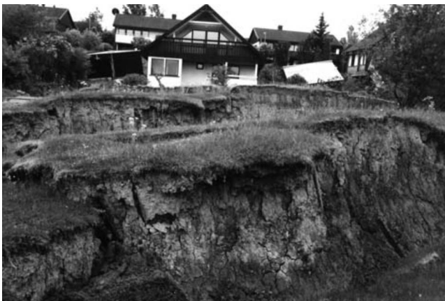
Fig. 7. Photograph of residential area in Vagnhäräd after slope failure within Trosa River Valley in 1997 (photographer: Jan Lindgren, Swedish Geotechnical Institute)
