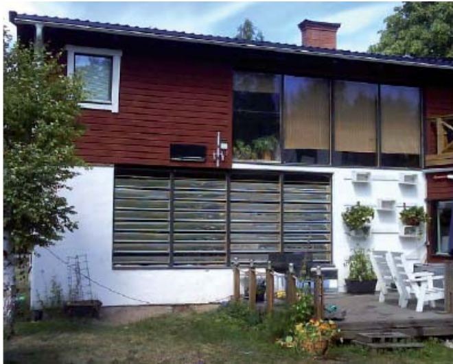
Figure 2.7 The Solgård solar window with the reflectors in a closed, vertical, position.
