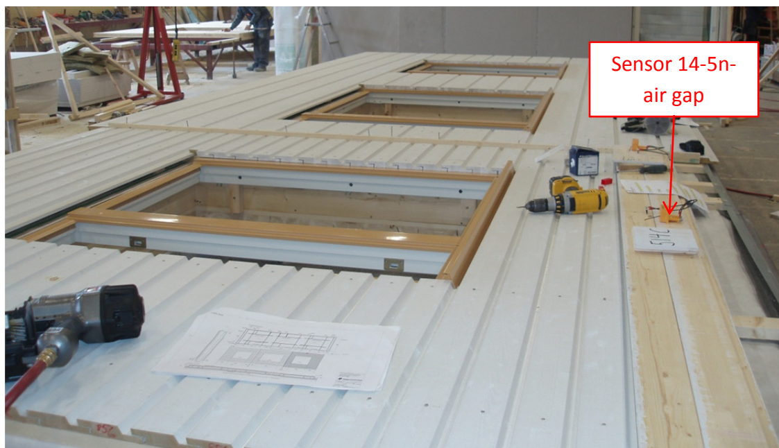
Figure 8.14-5n-air gap.2. Location of the studied position. Photo: SP Trä Skellefteå.
