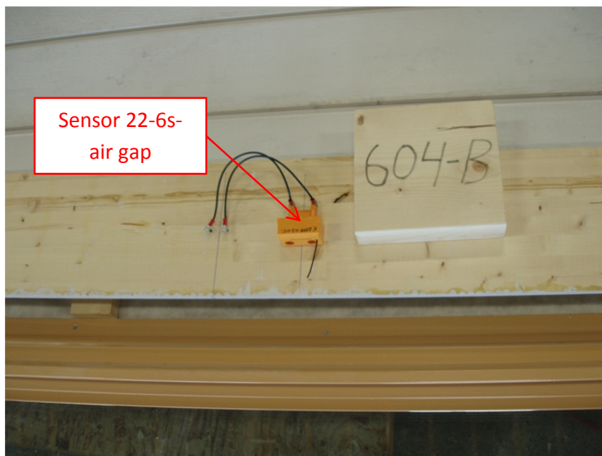
Figure 8.22-6s-air gap.2. Location of the studied position. Photo: SP Trä Skellefteå.
