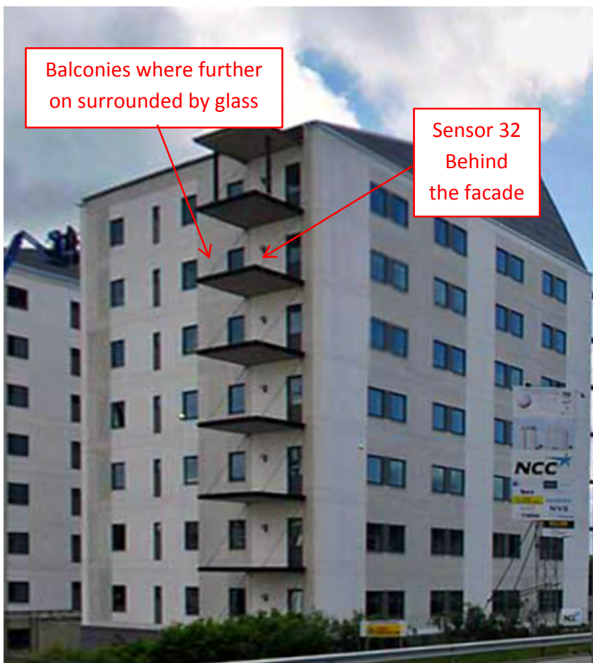
Figure 8.32.4. Location of the studied position. The balconies were further on surrounded by glass.
