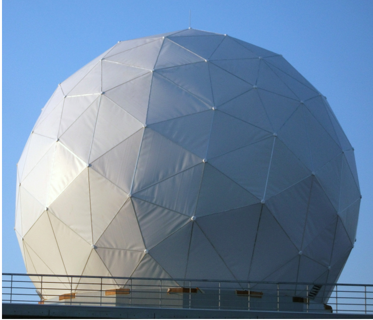
Figure 8: Photo of a metallic space frame radome protecting an antenna for satellite communications. The diameter is 13.7 m. Located at Chitose, Hokkaido, Japan. Photo courtesy of L-3 ESSCO Collins Limited.
