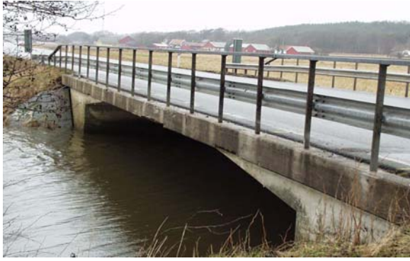
Fig. 6. Bridge N29 on Road Lv 845, Åskloster.
