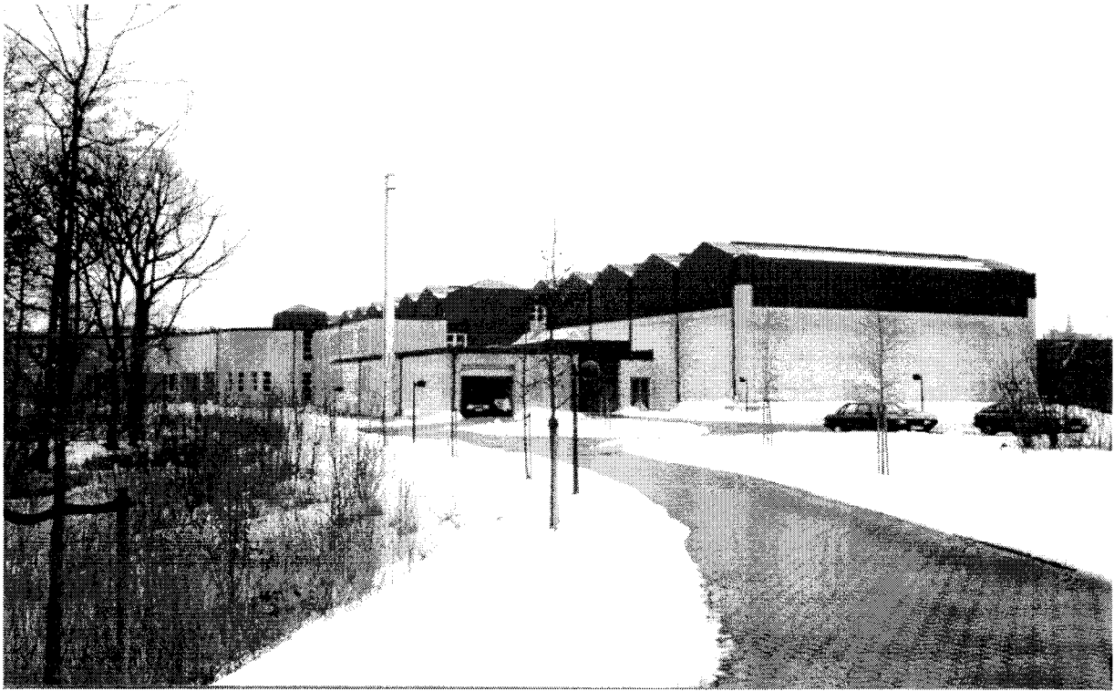
Figure 13 The repository building seen from the back.
