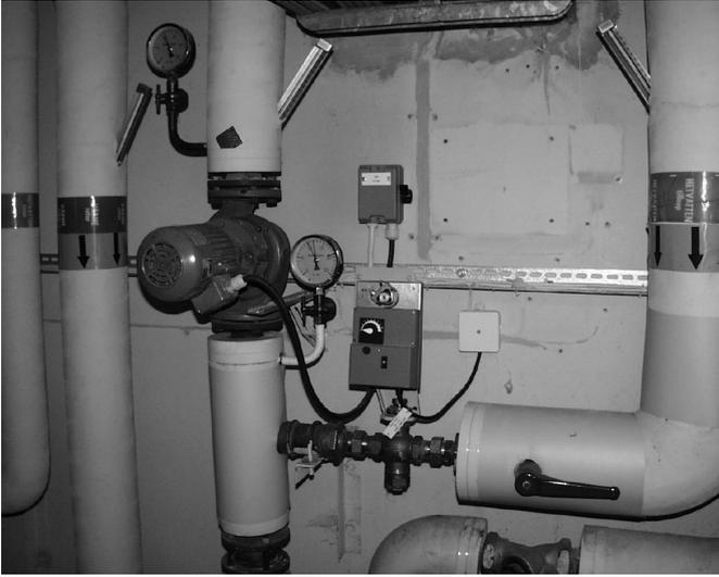
**Figure 5.** The control valve for the heating/ventilation system.
