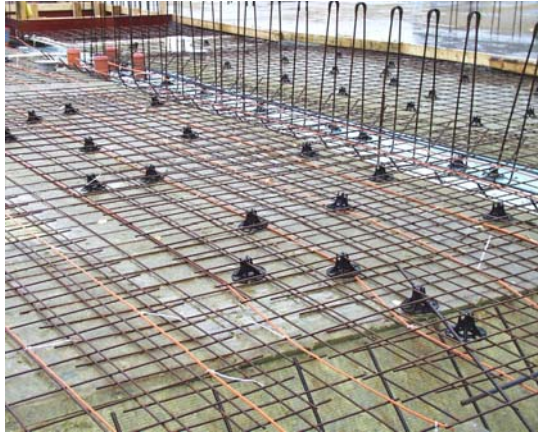
Figur 4.2 Elslingor i bottenplattan
