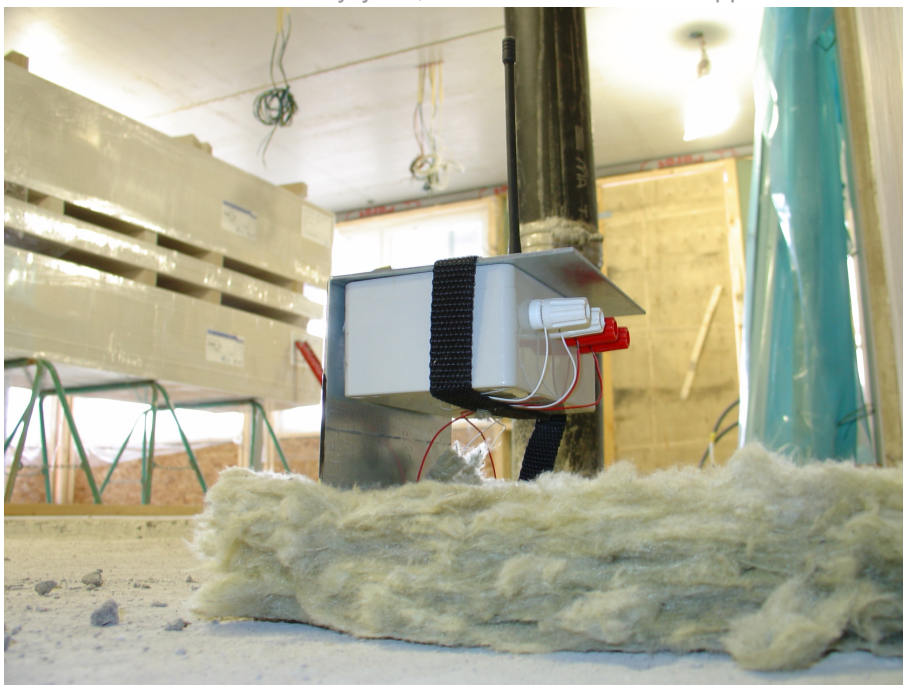
FIG. 2. Transmitter and insulation on top of concrete at the measuring position
