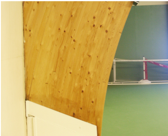
Figure 115-1. Arched column with steel parts (in white).
