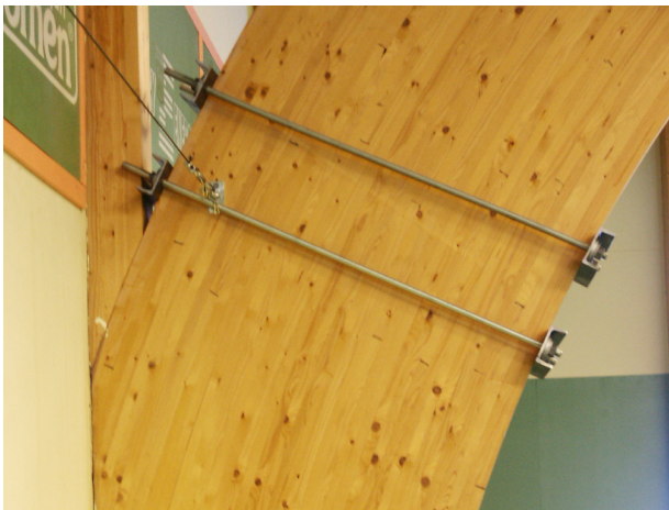
Figure 115-3. Temporary steel fixings attached to the column.
