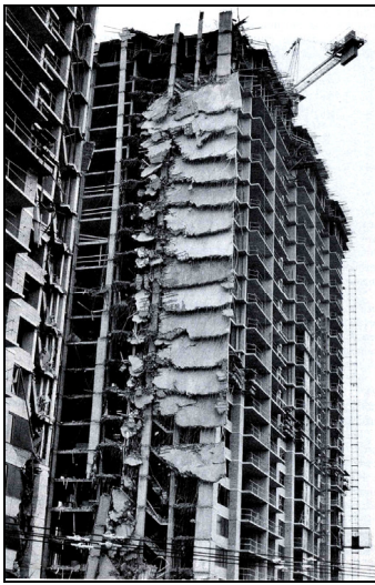
Fig. 4. Progressive failure of multi-storey concrete building due to premature removal of shoring, 1973, Virginia, USA.
