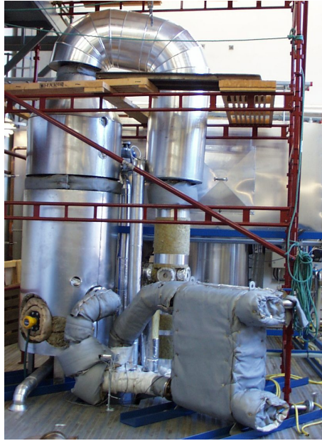
Figure 3.7: Installation of the plate heat exchanger aftercooler
