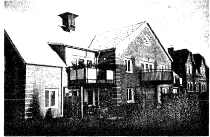
FIG. 4: An outline of the Malmö building. The framework is made of lightweight concrete and concrete.
