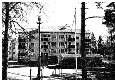
FIG. 7: An outline of the Stockholm building. The framework is made of steel columns and concrete.
