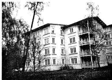
FIG. 6: An outline of the Växjö building. The framework is made of wood – quite an unusual solution for a four-storey multi-family building in Sweden.
