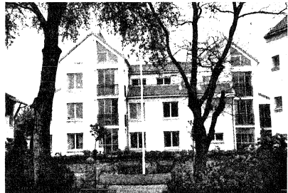
FIG. 5: An outline of the Helsingborg building. The framework is made of concrete.
